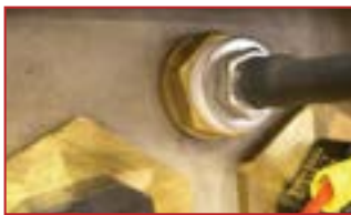
All sensing functions are integrated into one probe which can be replaced without draining the tank
